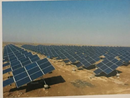
Installation Site: Xinjiang, China Project: 8MW Tilt Single Solar Tracker
