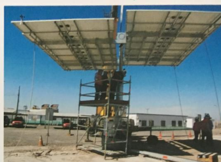
Installation Site: Chile Project: 20KW Double Axis Solar Tracker
