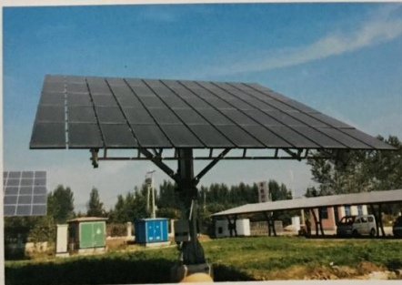
Installation Site: Shangdong, China Project: 7.8KW Double Axis Solar Tracker
