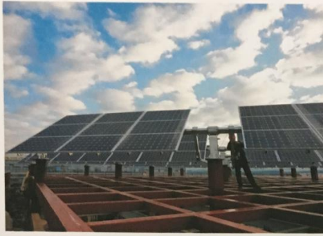
Installation Site: Yunnan, China Project: 900KW Roof Flat Single Axis Solar Tracker
