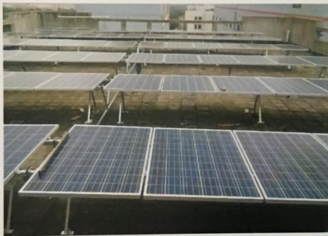
Installation Site: Zhejiang, China Project: 300KW Flat Single Axis Solar Tracker
