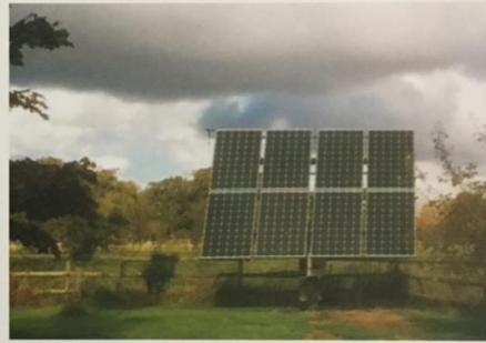
Installation Site: UK Project: 5.4KW Double Axis Solar Tracker
