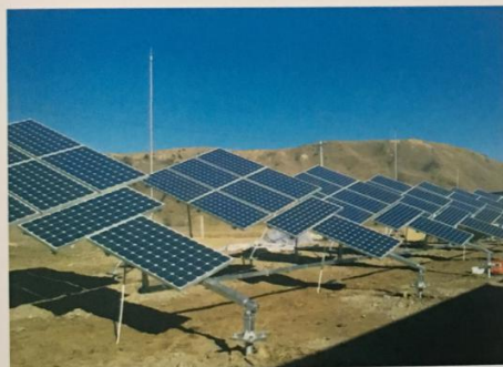
Installation Site: Sichuan, China Project: 4.8MW Tilt Single Axis Solar Tracker
