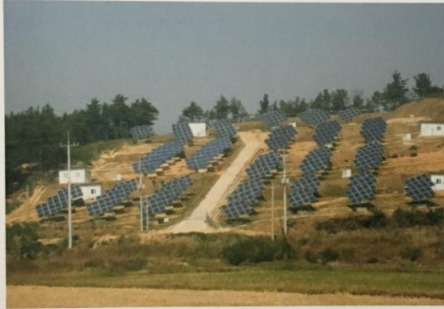
Installation Site: Shangdong, China Project: 4MW Double Axis Solar Tracker
