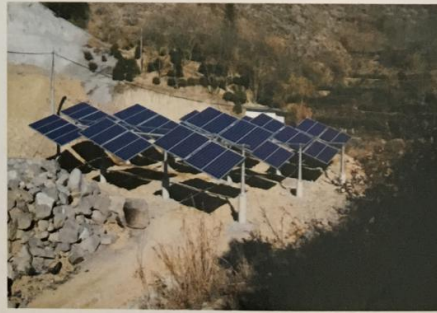
Installation Site: Lishui, China Project: 300KW Double Axis Solar Tracker
